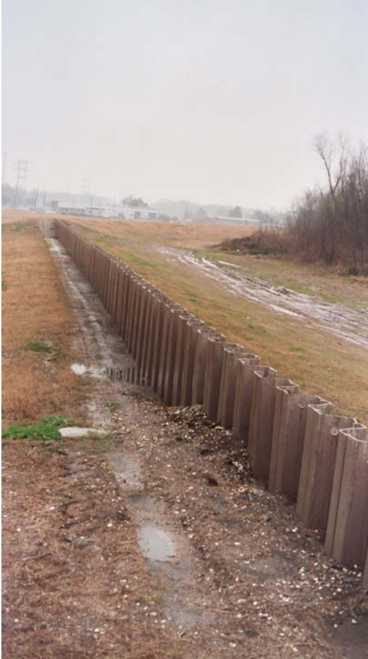
Figure 1 PVC sheet pile floodwall installed (Jan 98) in the town of Westwego, Jefferson Parish, LA
