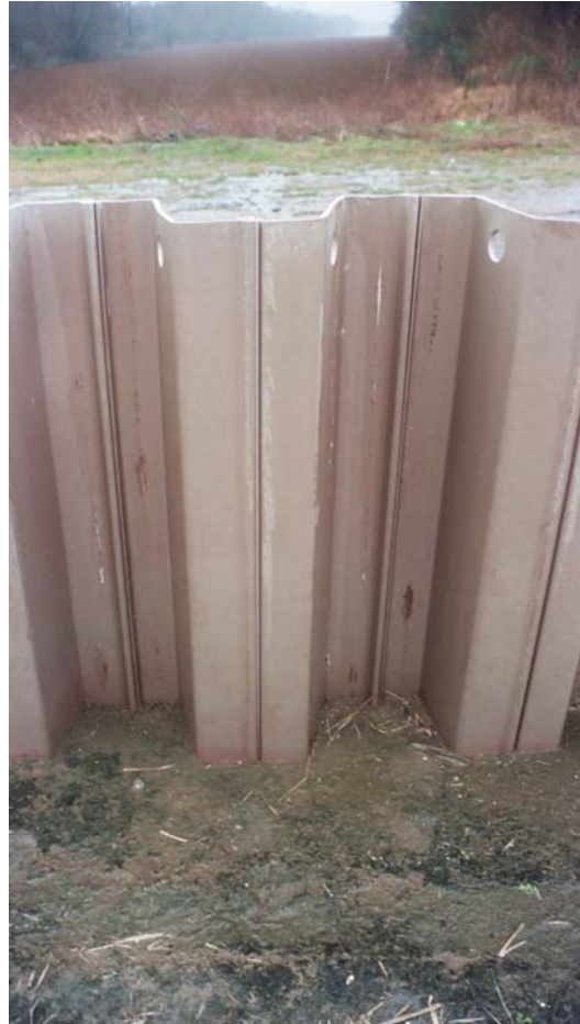
Figure 1 PVC sheet pile floodwall installed (Jan 98) in the town of Westwego, Jefferson Parish, LA
